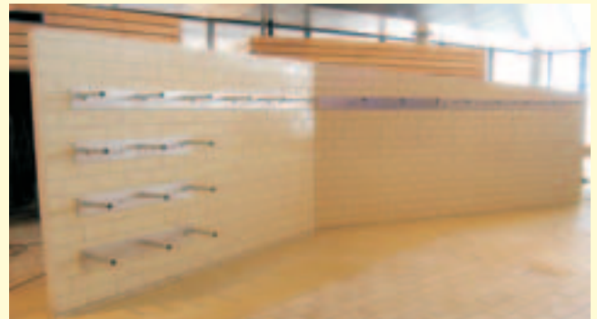
Towel hooks on a wall with tiles blocking the visibility behind.
